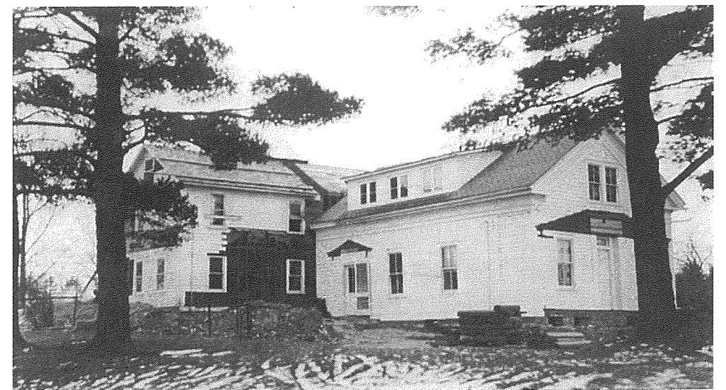
THE OLD WEST DISTRICT SCHOOL HOUSE AS IT WAS BEING ATTACHED TO BROOKSIDE FARM COTTAGE, NOW THE RESIDENCE OF MR. AND MRS. JOHN FRASER, 95 DEVON ROAD.
