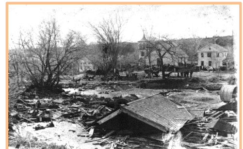
Chapel Street, East Lee, after the 1886 flood.
